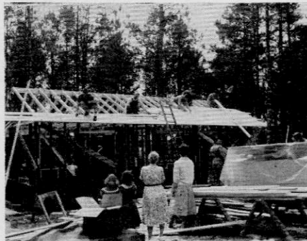
Starting sheathing on roof. Weatherboarding below.
