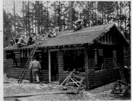
Shingles on the Roof. Siding finished.
