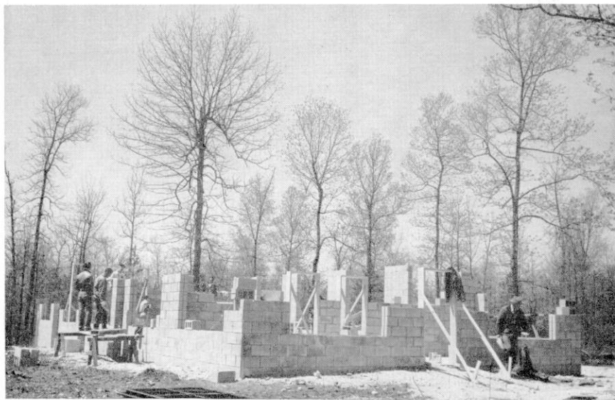
Madison College students erecting Industrial Arts Building
