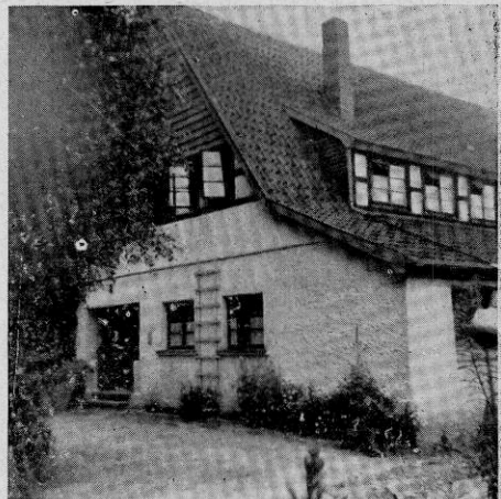
A finished dwelling of mud brick construction
