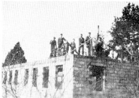
Construction of Wood Workshop and Students and Teachers at Work
