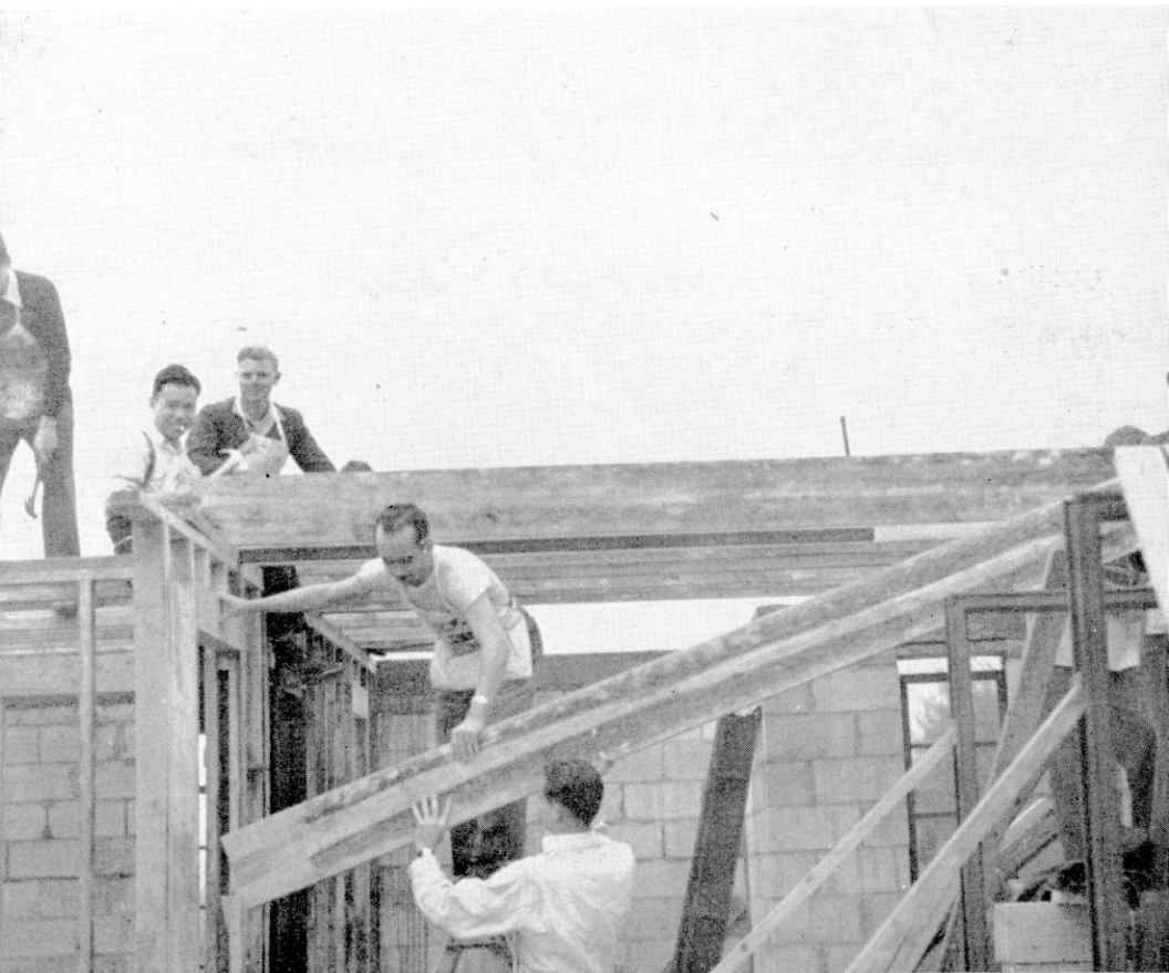
Carpentry Class Helping Build Apartment House
