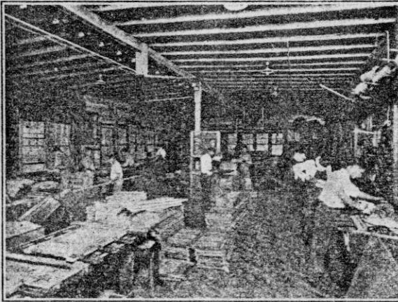
Preparing Building Material
