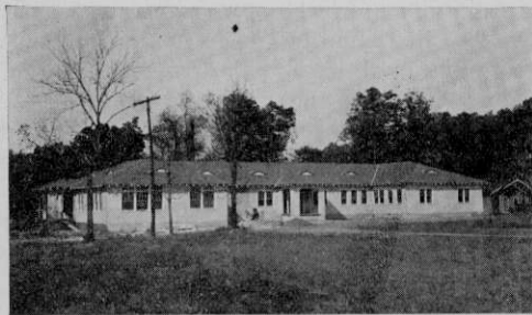
The building as it now appears
