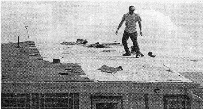
Installing a new roof
