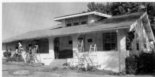
The Heritage House painting underway
