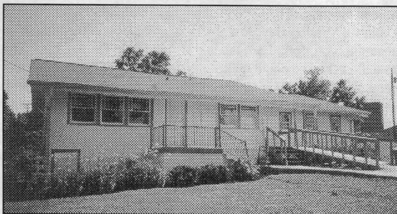
Rear of Heritage House.
