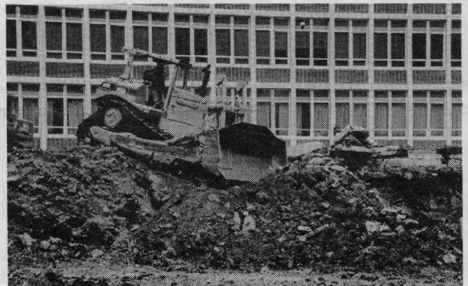
Digging out the fountain.
