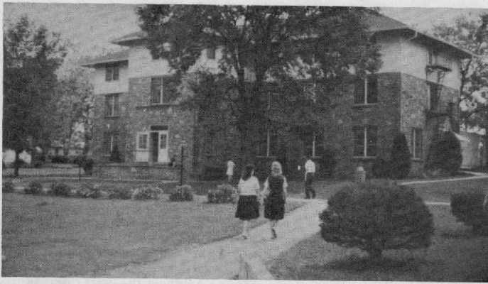
Williams Hall, built by students and faculty, served as a dormitory for Madison College young women from 1941 to 1964, and for a time as an academy dormitory. It was demolished in early December, 1976.
