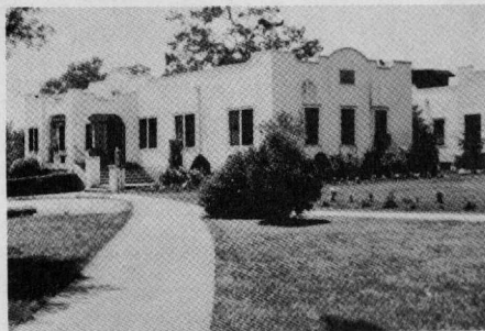
Administration building (for both college and hospital) constructed in 1928.
