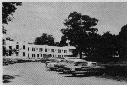
Surgical & Obstetrical Wing completed in 1938.
