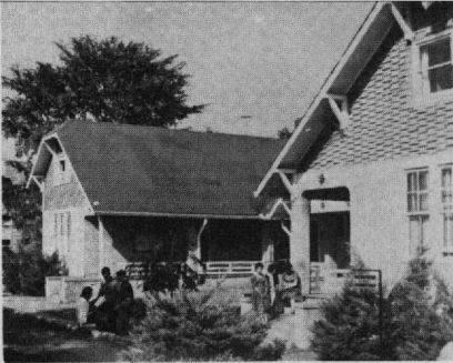
Helen Funk Assembly Hall, removed in July, 1975. Built in 1922, it was one of the four large buildings on campus. It had three floors and was used for various purposes—library, chapel, administrative offices, dormitory, Dorcas, pastor's study, alumni office, etc.
