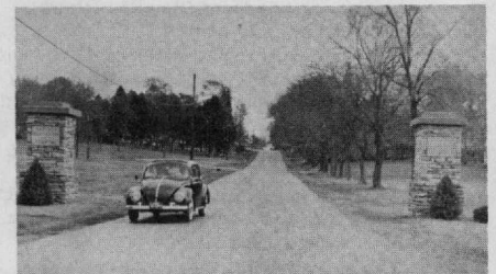
The pillars at the Larkin Springs entrance to Madison Hospital, a gift of the class of '43, were pulled out shortly before Homecoming, due to widening the road. The plaques, with their inscriptions--Madison College on one and Madison Sanitarium and Hospital on the other, and the year built--were saved. Another landmark gone.
