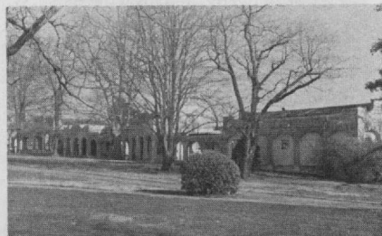
Old San General, the last of the original small cottages built about 1908, the beginning of Madison Sanitarium and Hospital, was demolished shortly before Homecoming in June, 1975. Sorry we didn't have a better black and white picture
