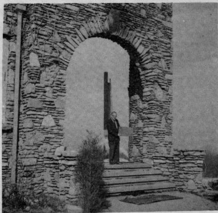
W. A. Sowers, academy principal, standing at entrance of burned out Science Building, holding rescued plaque which read, "Floyd Burton Bralliar Memorial Hall, Erected 1933." (Smokestacks of Central Heat may be seen through the open doorway).
