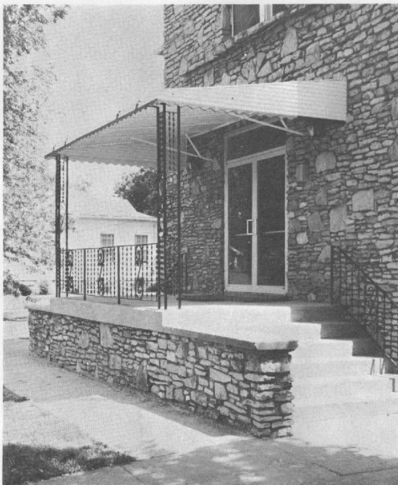
New, attractive entrance and foyer to Williams Hall, showing aluminum-framed glass doors, protective canopy, wrought-iron railings.
