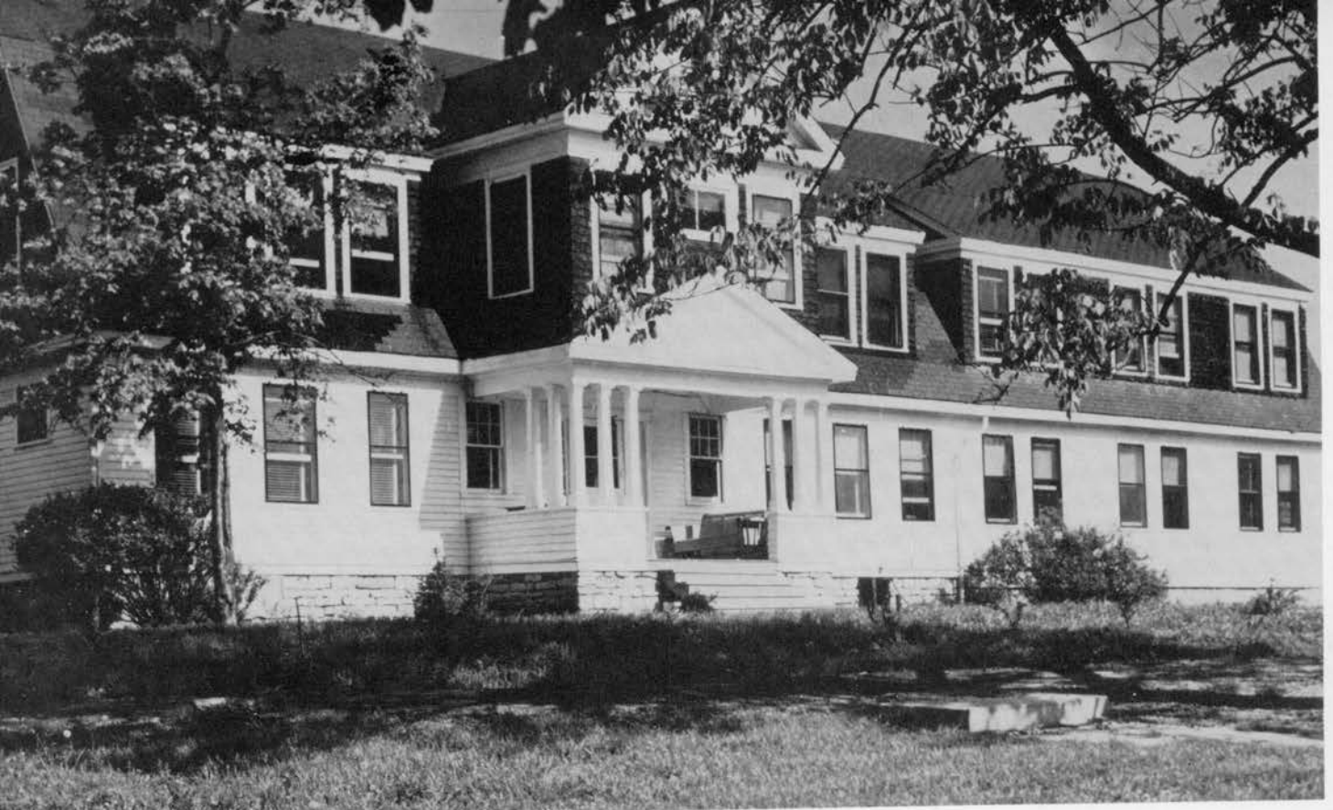
Gotzian Home - Men's Dormitory
