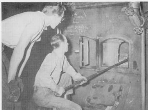
Students look forward to their certificate after completion of a one-year intensive course including Heating Plant Operation, Plumbing, and Basic Electricity.
