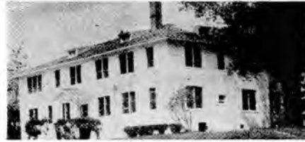
Forsyth Memorial Sanitarium Tallahassee, Florida
